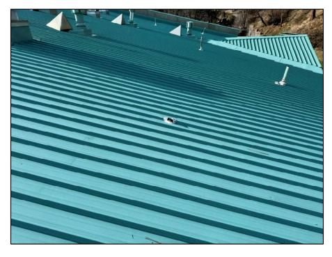
Loyalton report photo, dated January 6, 2025, of bent and/or deformed ribs at the east side of the easternmost dormer at the north side of the roof.
