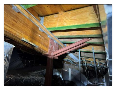
There were dark stains on the roof sheathing at the locations of the displaced roof vents above.
