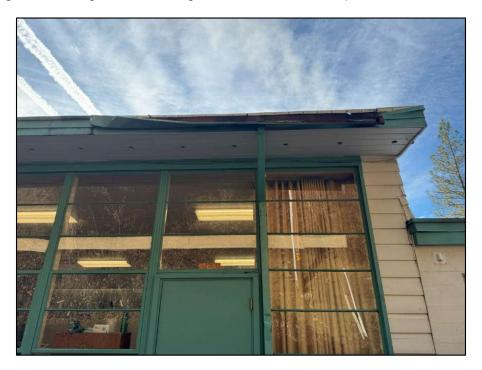
There was a separation in the metal flashing at the roof edge above the window.
