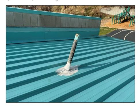
There were gaps with rounded, oxidized edges in the sealant applied around the roof vent at the east side of the south roof facet.
