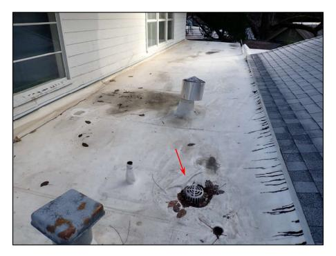
There were dark stains on the roofing membrane around the roof drains at the building's south hallway.
